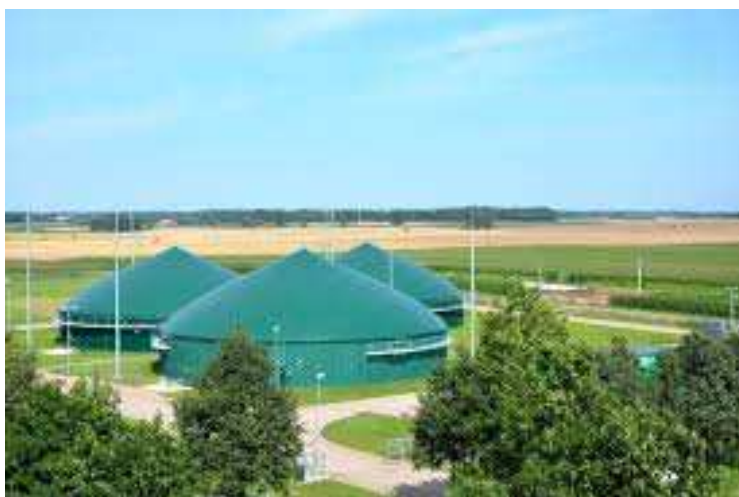
Fig. 5.7. Fermentation tanks in an agricultural biogas plant – view of the fermentation tanks ( https://poranny.pl/biogazownia-w-rybolach-pracuje-juz-pelna-para/ar/10183410 )
